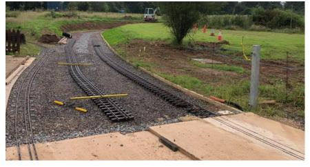
Work has also continued in areas around the track bed and we now have the section curving from the level crossing to the top of the site looking almost complete. With expertly graded sides, subbase and concrete edging in place to retain the ballast we will shortly be starting to lay track in this section. A real milestone to have reached and one to be rightly proud of.
