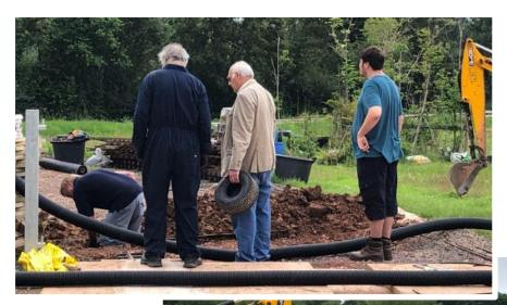
In order to provide power to our donated signal box a trench (yes another trench!) has been dug next to the level crossing and ducking laid for power cables, with a spare duct should we need to cross under the track in the future! Work in progress on a very hot day below.
