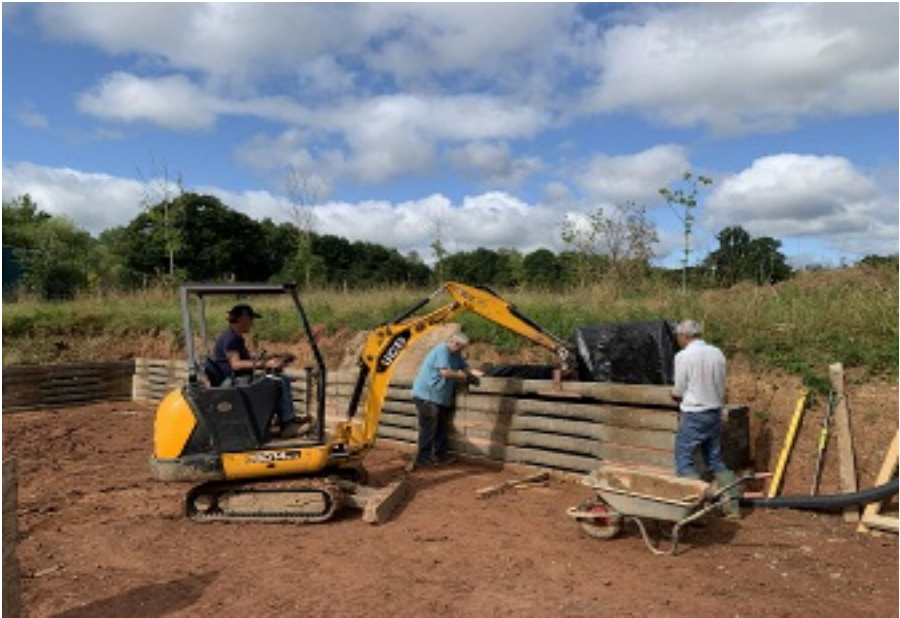
Setting the last ex BR sleeper in the yard retaining wall
