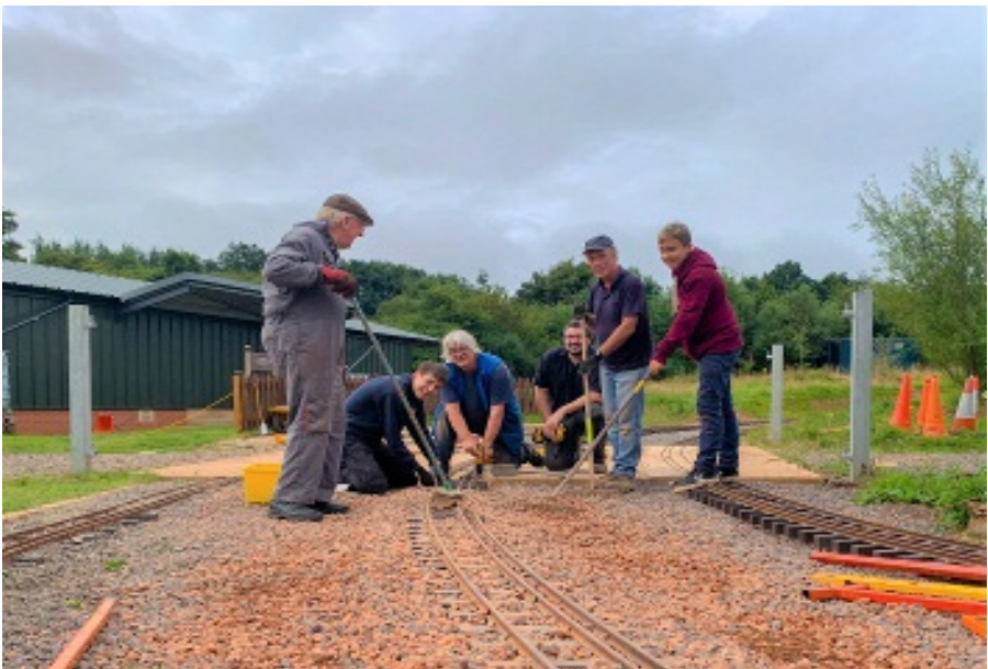
Track laying at West Buckland
