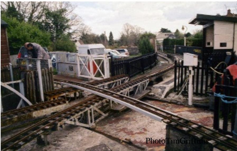
A most striking part of the track is the pneumatically operated traverser for gaining access to the running track from the team ing bays. This obviously took some engineering, but was well thought out and worked extremely well. (The lift out section, which hgives accessto the car park, is in place in the picture. Ed)
