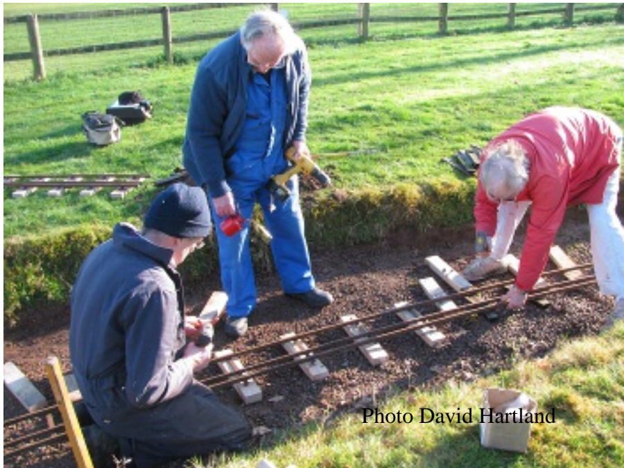
Members of the "track gang" relaying the track in the cutting
