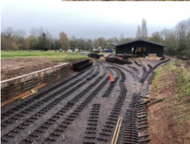
The marshalling yard takes shape.
