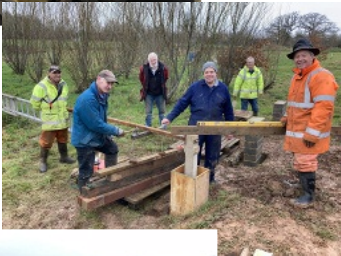
First pier on the elevated track
