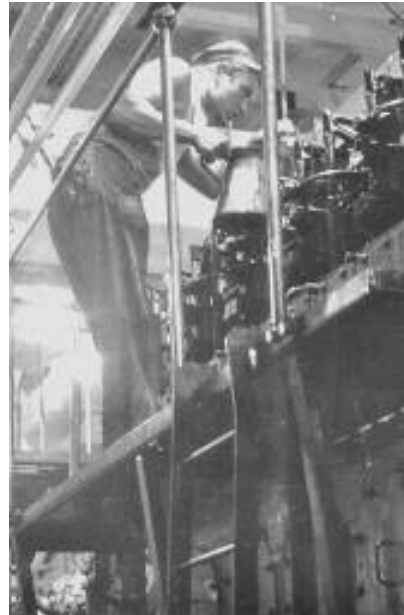
Oiling the rockers.
